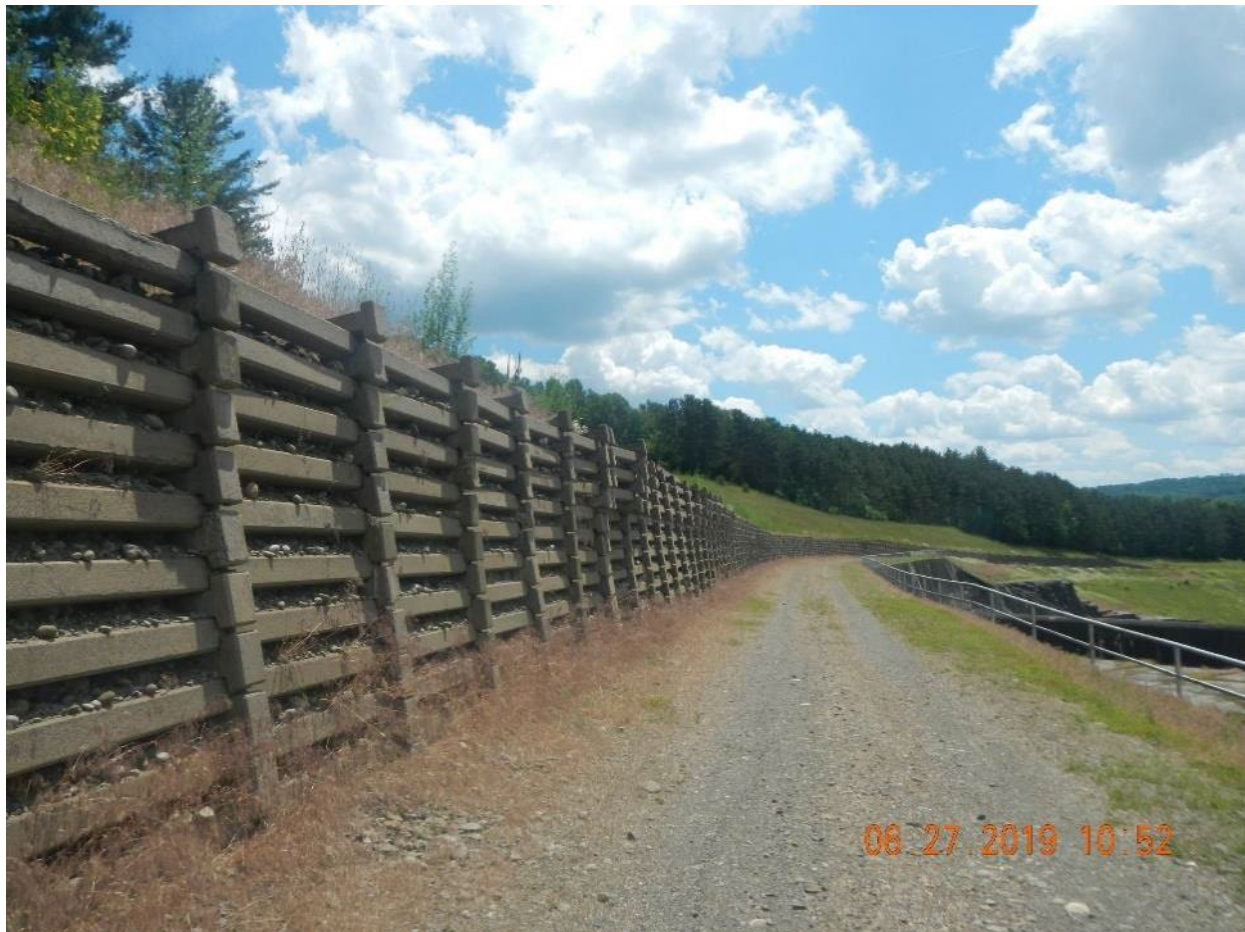
Figure 1-2 Crib wall and adjacent gravel maintenance road (Prospect Street).
