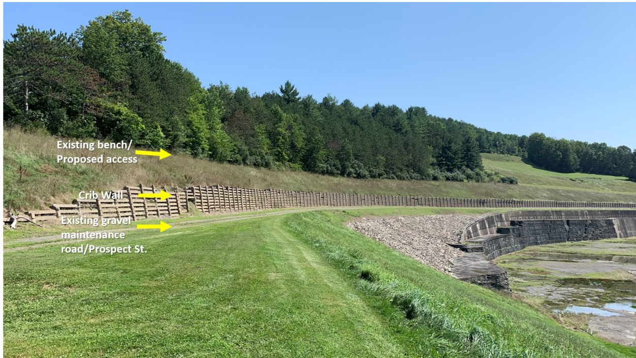
Figure 1-3 Photo showing locations of the existing maintenance road, crib wall, and existing bench/proposed access.
